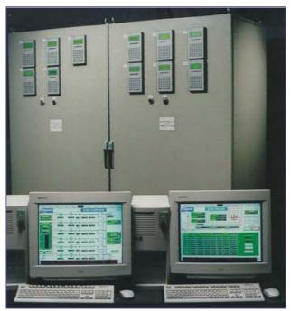
Installation of flow computers communicating to a PLC sysytem within a control room environment.
